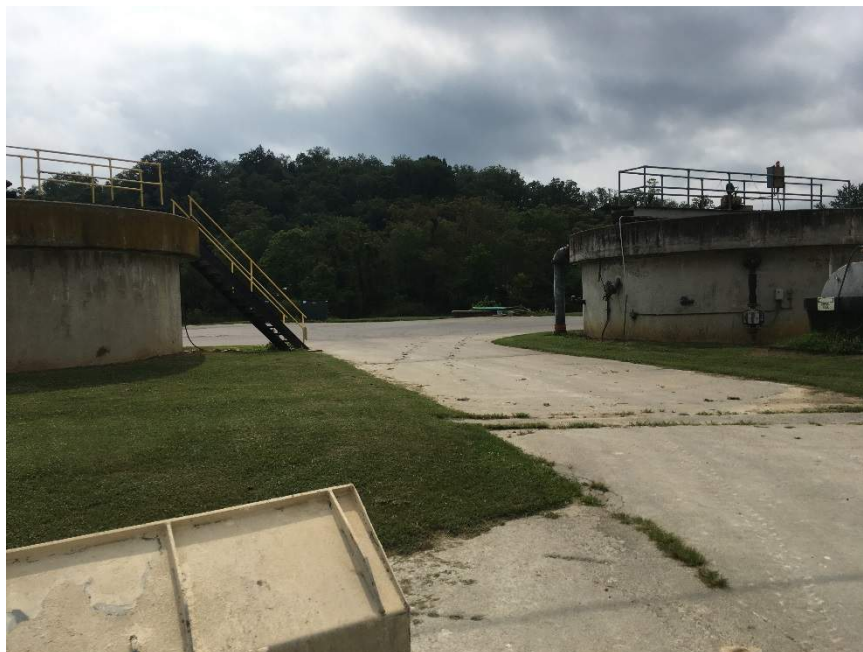
Figure 28. Sludge thickener structures. Concrete is in generally good condition.
