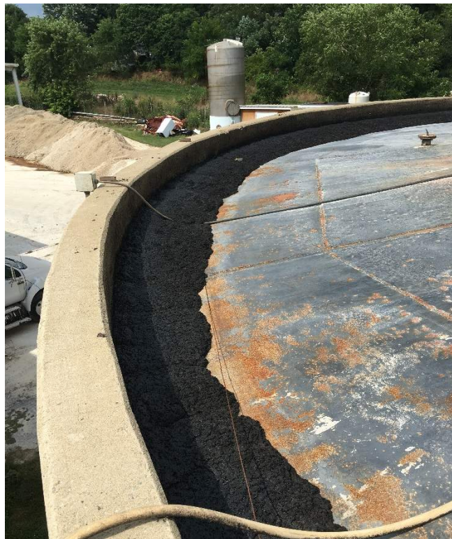
Figure 26. Exterior concrete wall and steel-clad roof of digester.
