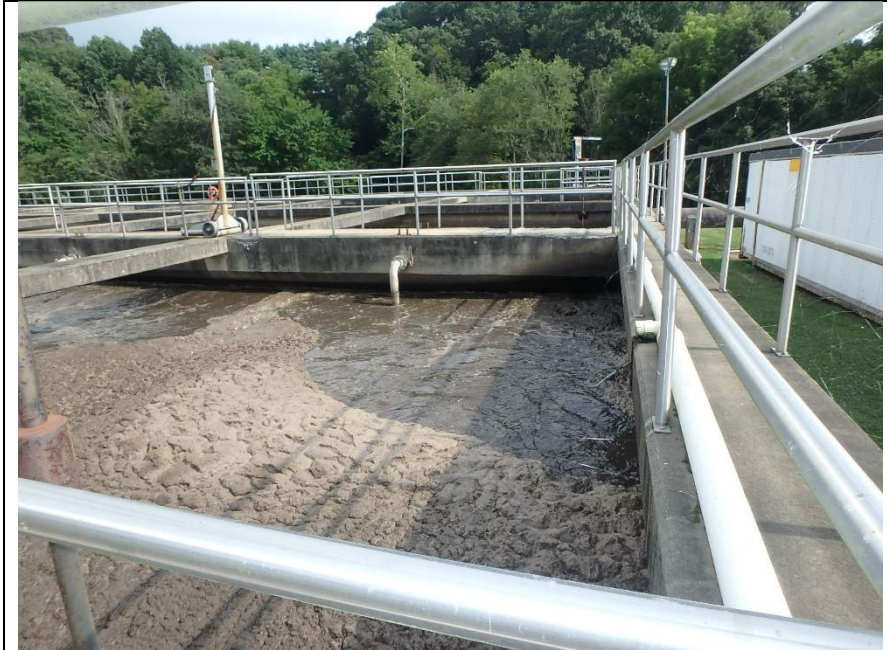
Figure 11. Concrete at aeration basin is in generally good condition.
