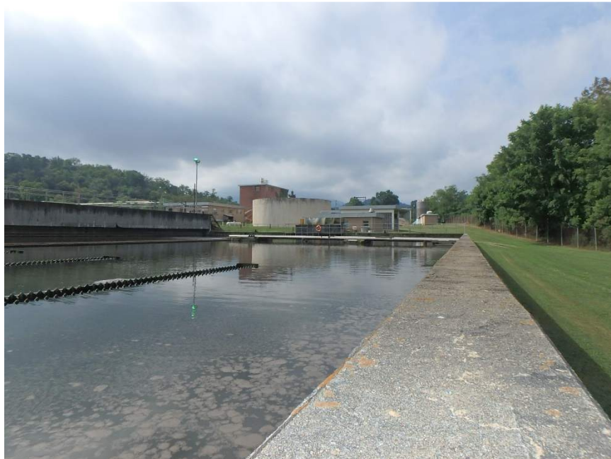
Figure 20. Concrete at secondary clarifier is in generally good condition.
