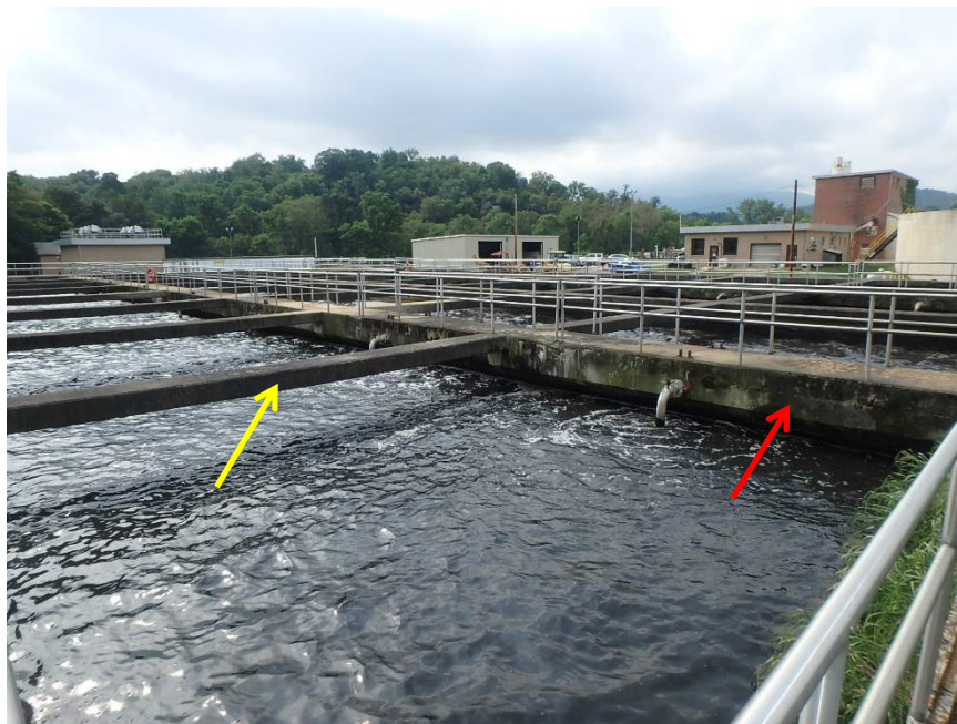
Figure 8. Aeration basin. Walkway (red arrow) tops interior wall that separates chambers. Horizontal braces (yellow arrow) provide lateral stability to walls.
